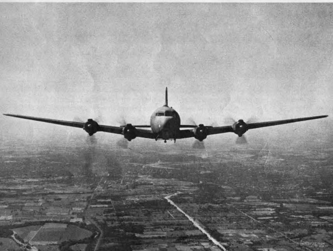
DIHEDRAL EXTENDING FROM ROOTS DISTINGUISHES C-54 HEAD-ON. NOTE CIRCULAR FUSELAGE
